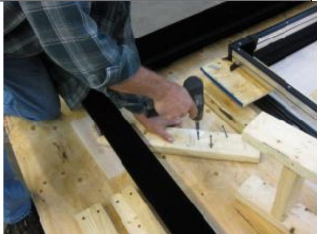
7) Remove the block-fastened components using a cordless drill.
