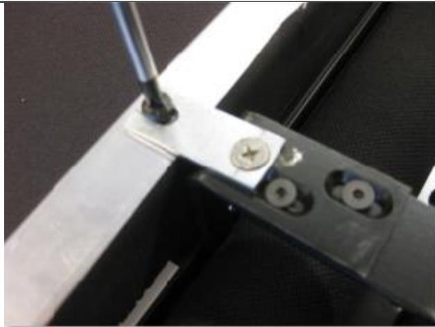
31) Simply turn the bracket into position and insert the black pan-head screw as shown.
