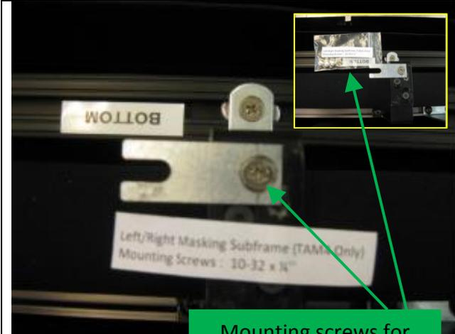
Mounting screws for screen subframe installation.
