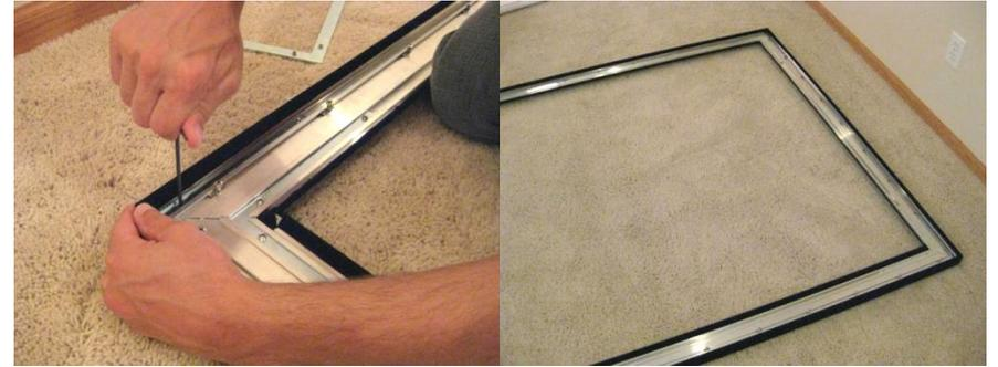
**Install Last Short Side.** For this fourth piece, a short side, insert its L-brackets but do not tighten at this time. Align the four L-brackets into their mating slots into the top and bottom frame pieces and slide into position.
