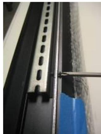
Mark where your DIN rail bar is to be mounted to the ceiling joists. Install using the included SS screws (or your substitute). At least three screws, securely mounted into your joists, are required. If you have a very curvy ceiling, you can space out a screw or two with washers. You don't want the DIN rail to be curvy, or else the case won't engage all the way.
