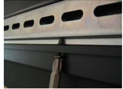
2) Locate the bag in the white remote box that has the five stainless steel truss head screws. Use a spirit level and mount the DIN rail to your wall using these screws. If you have a very curvy wall, you can space out a screw or two with washers or shims. You don't want the DIN rail to be curvy, or else the case won't engage all the way. Make sure at least three screws are securely mounted into a stud.
